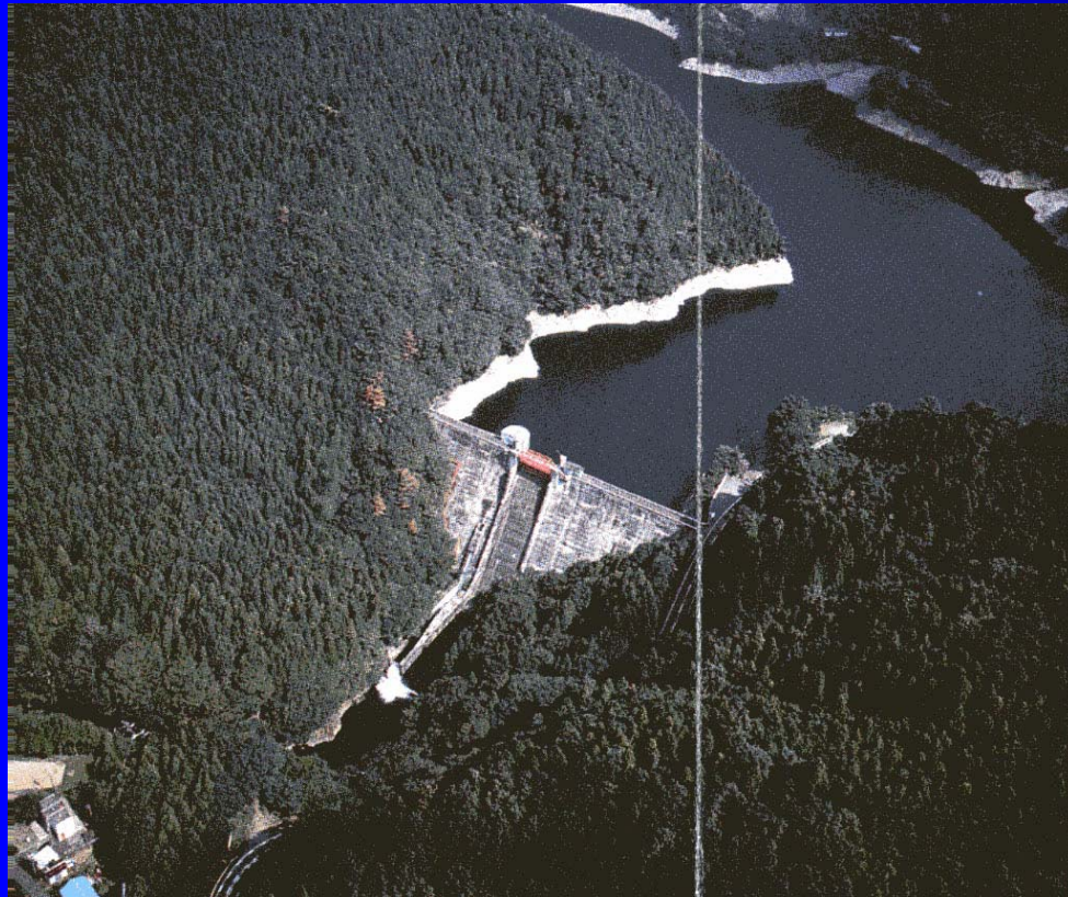
Yasu River Dam
