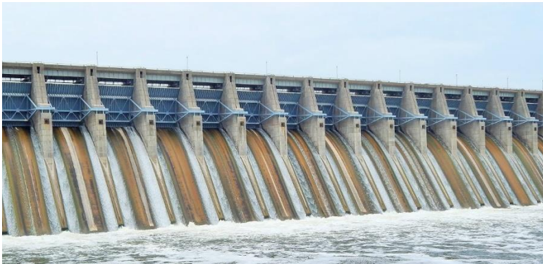
Whitney Lake Dam – USACE SWF District
