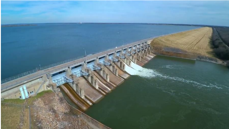
Lavon Lake Dam – USACE SWF District
